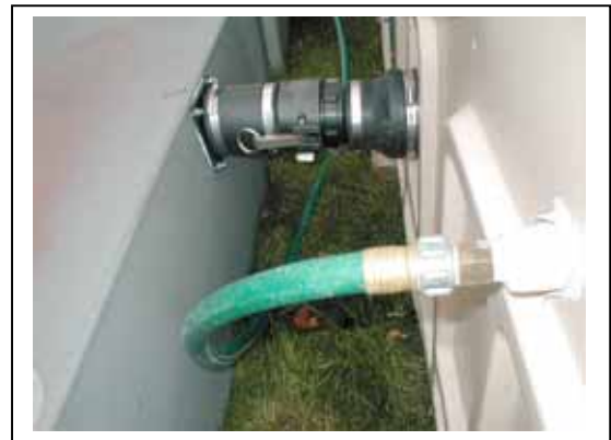
Water and Sewer Connection
